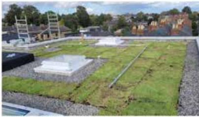
Unlike conventional roofs that drain water quickly, blue roofs slow stormwater runoff. Image: ACO
